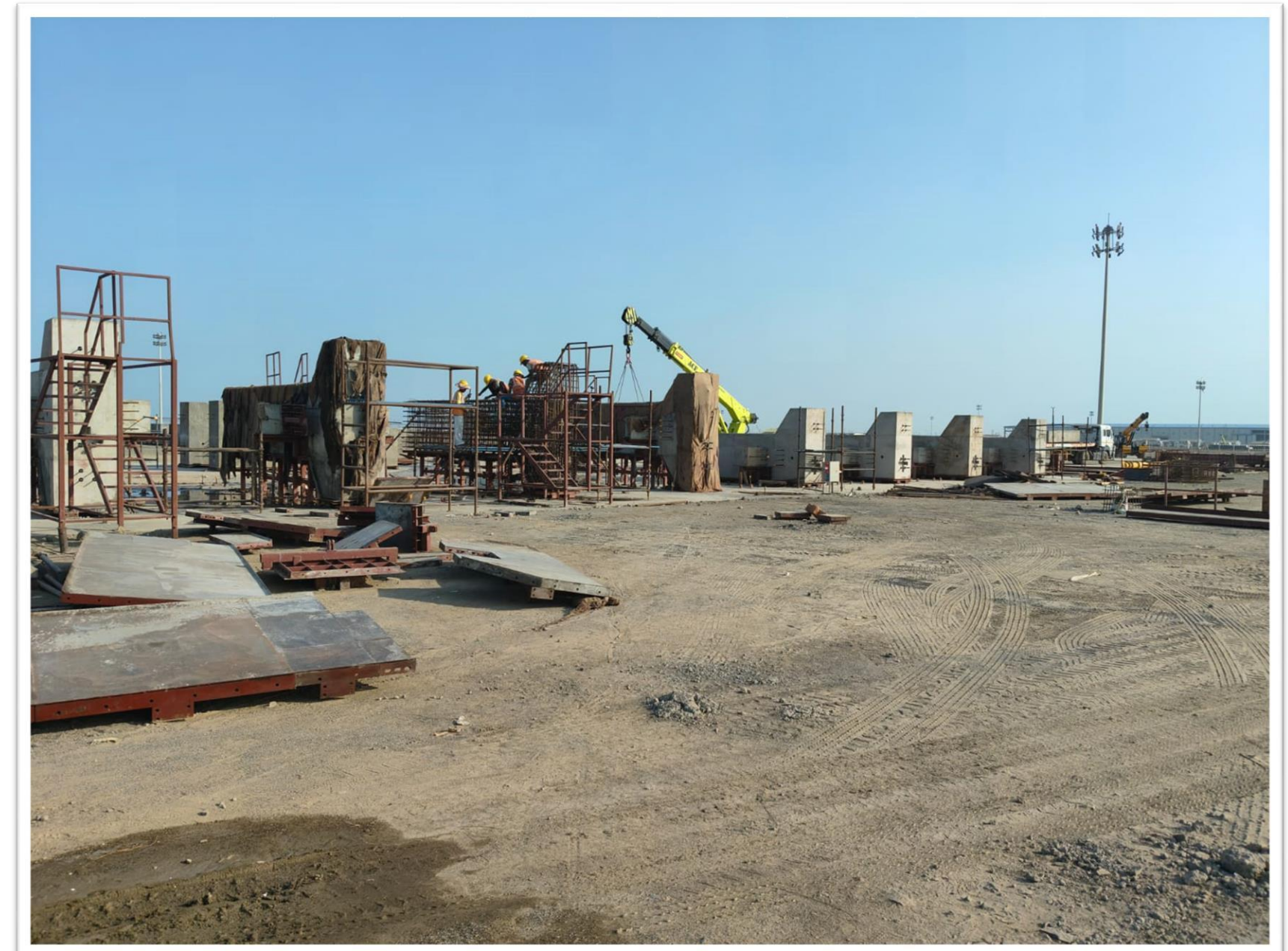
ADANI MUNDRA PETROCHEMICAL 100 CUM CONCRETING PER DAY
