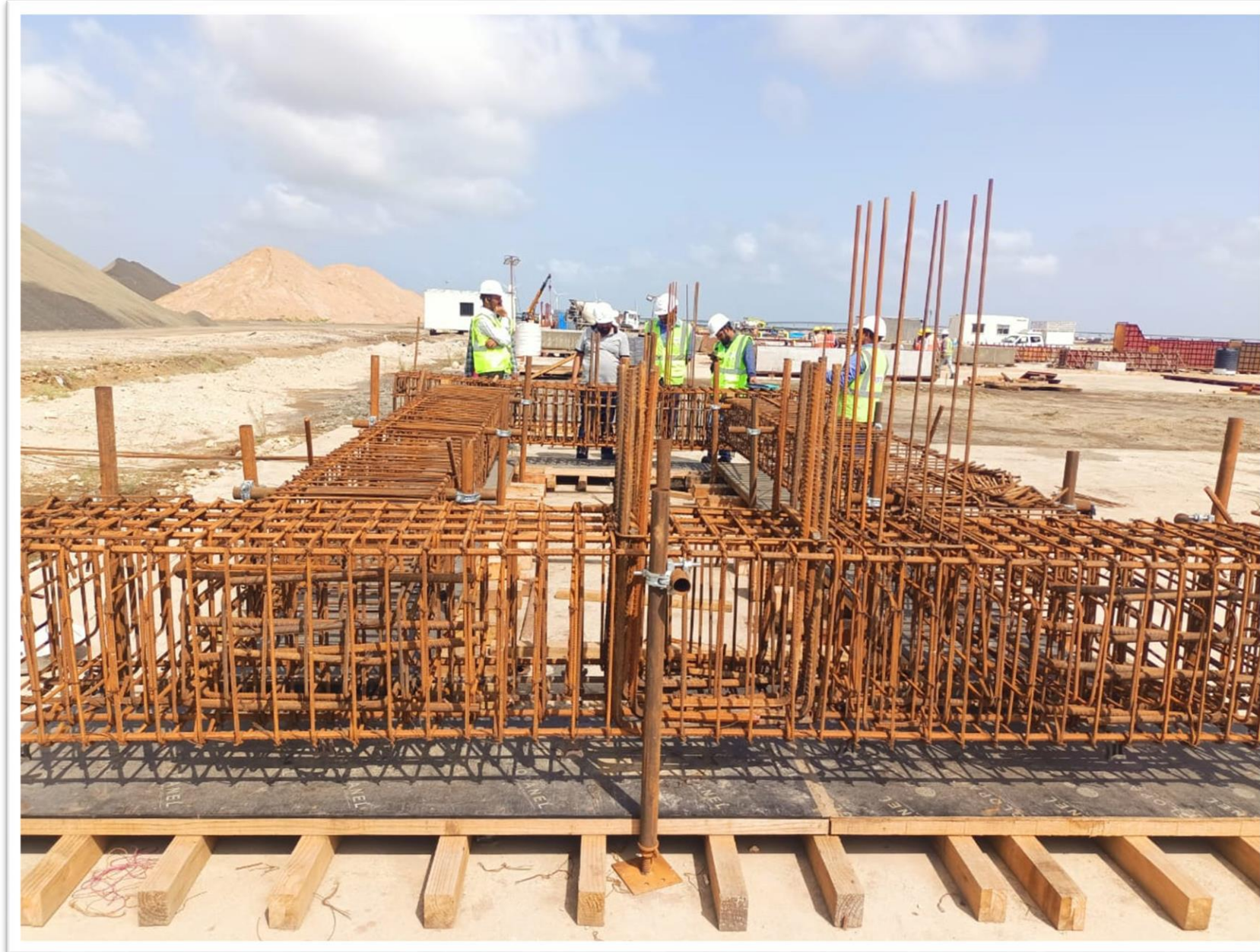
6 MTR H FRAME WITH M50 CONCRETE
